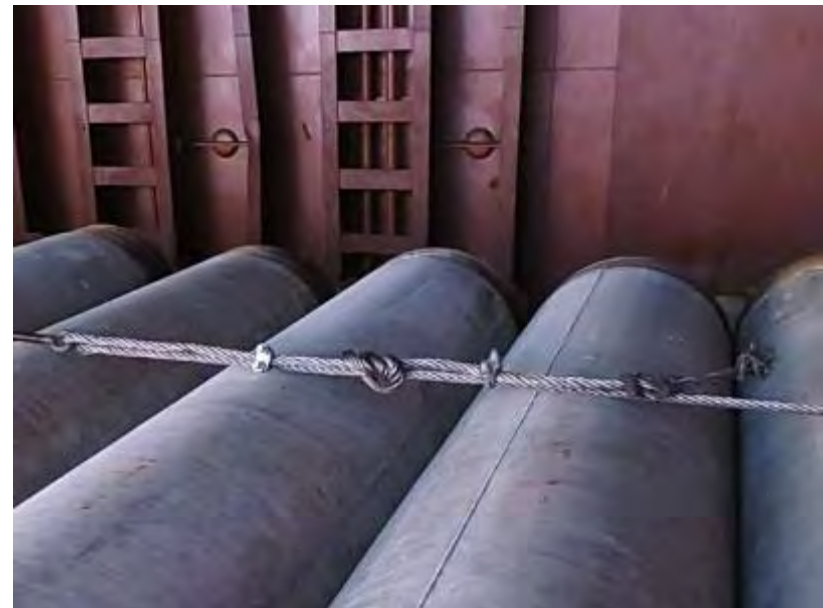
Incorrect way of connecting two wires and using bulldog grips. Insufficient number of grips used.
