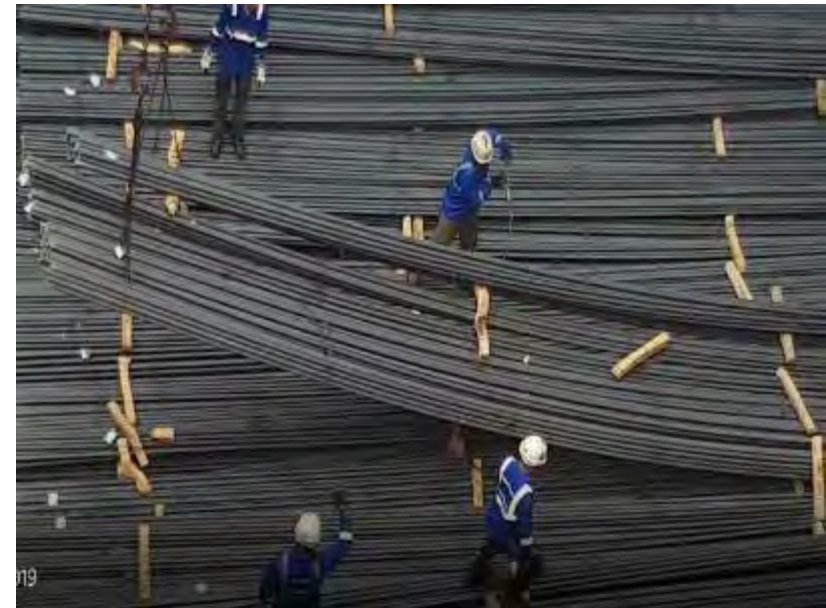
Tip-lifting technique used for off-loading rebars.
