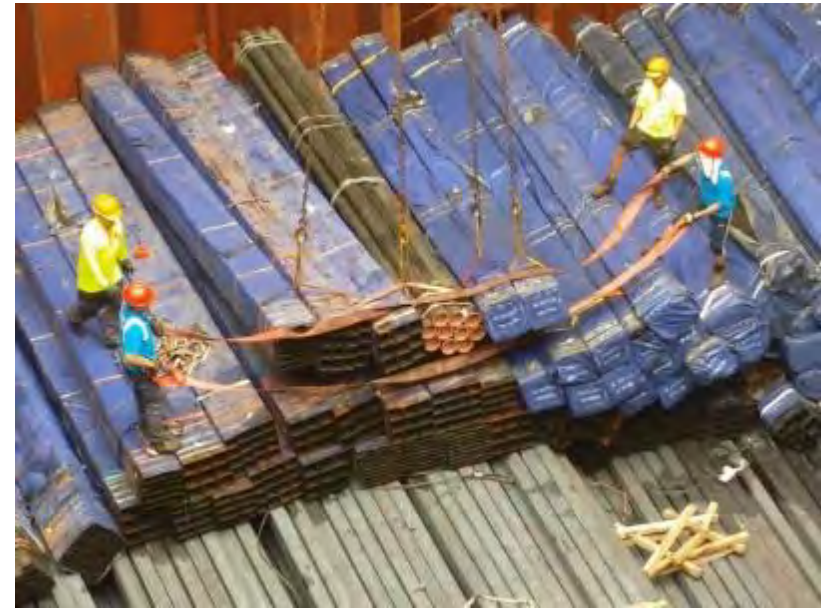
Sorting hooks used to tilt the pipes to allow for the passing underneath of the nylon lifting straps.
