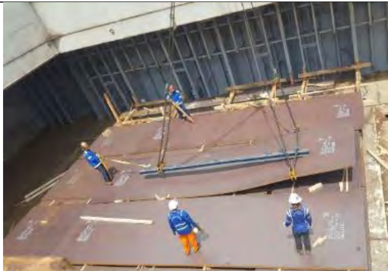
Off-loading of unbundled, unpacked steel plates. Use of 'C' hooks and a spreader.
