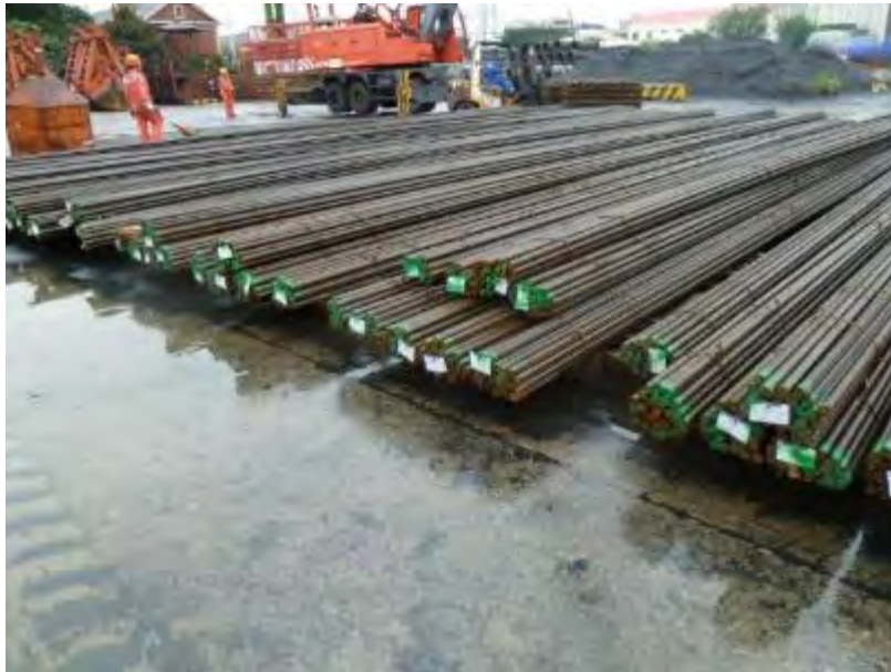
Rebar in open storage prior to shipment showing signs of corrosion.
