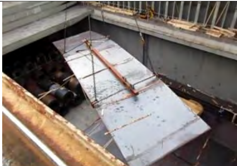
Off-loading of unbundled, unpacked steel plates. Use of 'C' hooks and a spreader.
