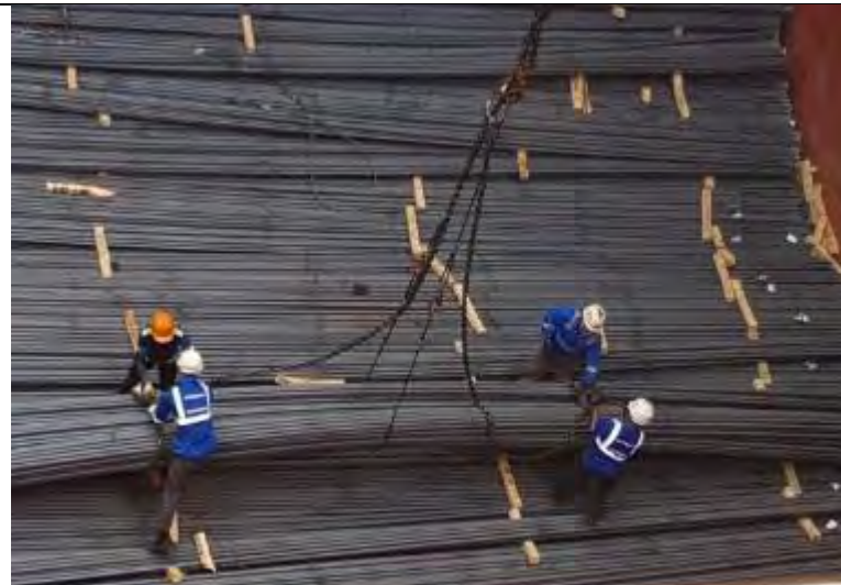
Lifting the middle part of the rebar bundle with the use of a wire, to pass the choke hitch sling. The dunnage assists in passing the lifting wire.
