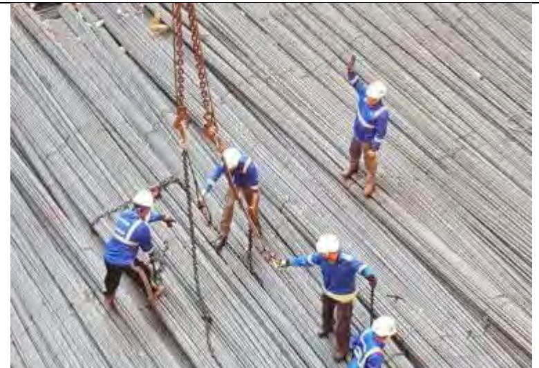
Once the lifting chains are in place, the short wires are removed.
