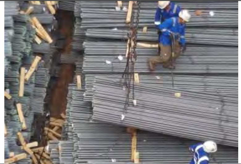
Tip-lifting from the end of the rebar bundles.
