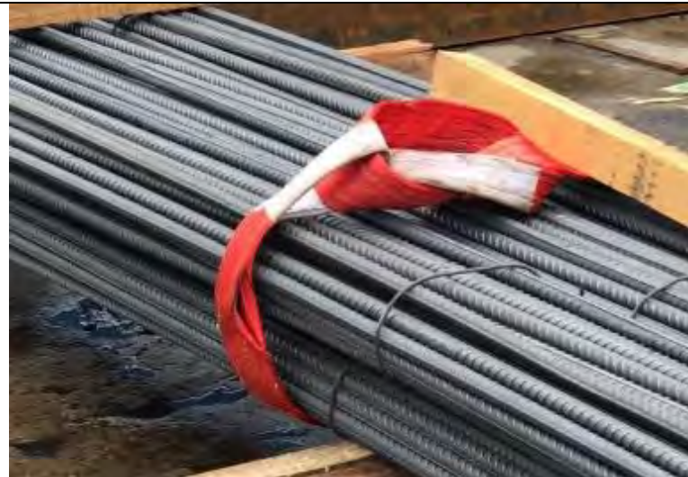
A sling combining six bundles of rebars ready for loading.
