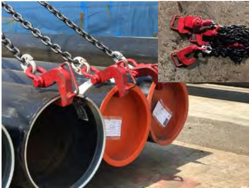
Using pipe hooks for the discharge of 12" open joint steel pipe.
